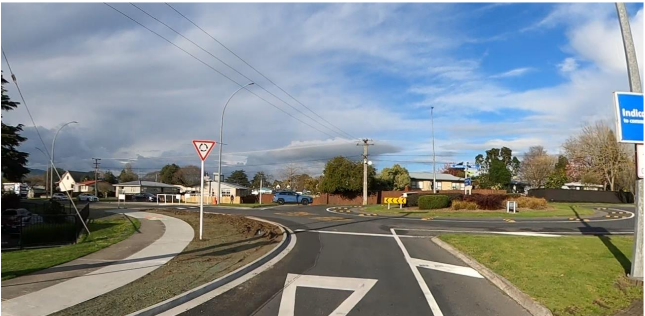
Figure 5: Shakespeare Street/Cook Street Roundabout: Post-Construction
