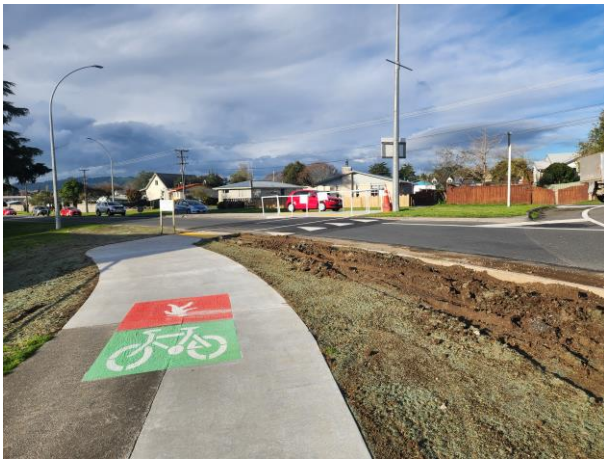
Figure 9: One vehicle space allowed before or after the Swedish-styled pedestrian crossing point on the northern approach of the roundabout
