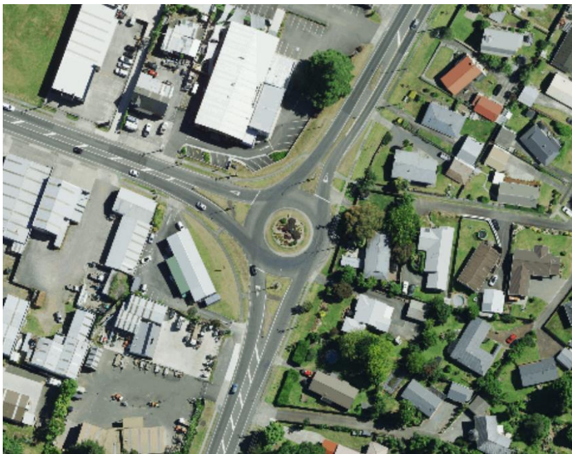
Figure 4: Shakespeare Street/Cook Street Roundabout: Pre-Construction
