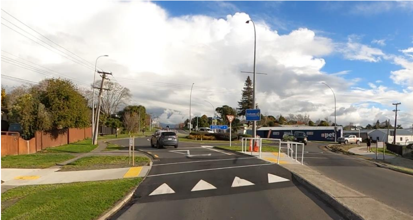
Figure 8: Swedish-Styled pedestrian crossing point Swedish-styled pedestrian crossing point on the northern approach of the roundabout
