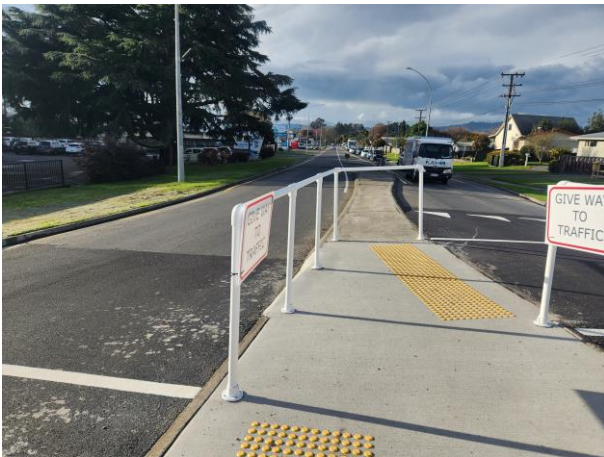
Figure 10: Widened traffic median island with pedestrian fence for the Swedish-styled pedestrian crossing point on the northern approach of the roundabout
