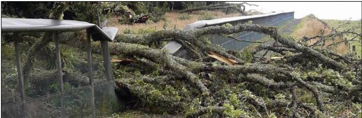
Figure 2: Tree fall causing a fence breach and cleaning up the fall
