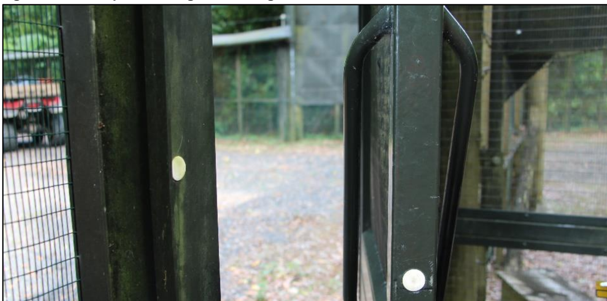
Figure 6: A pedestrian gate showing the location of the two reed switches
