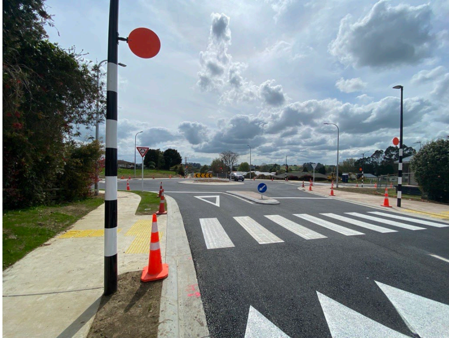
Rolleston Street view of the new roundabout
