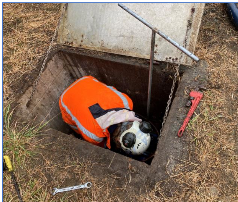
Shutting off Valves – Bridgman Road Site
