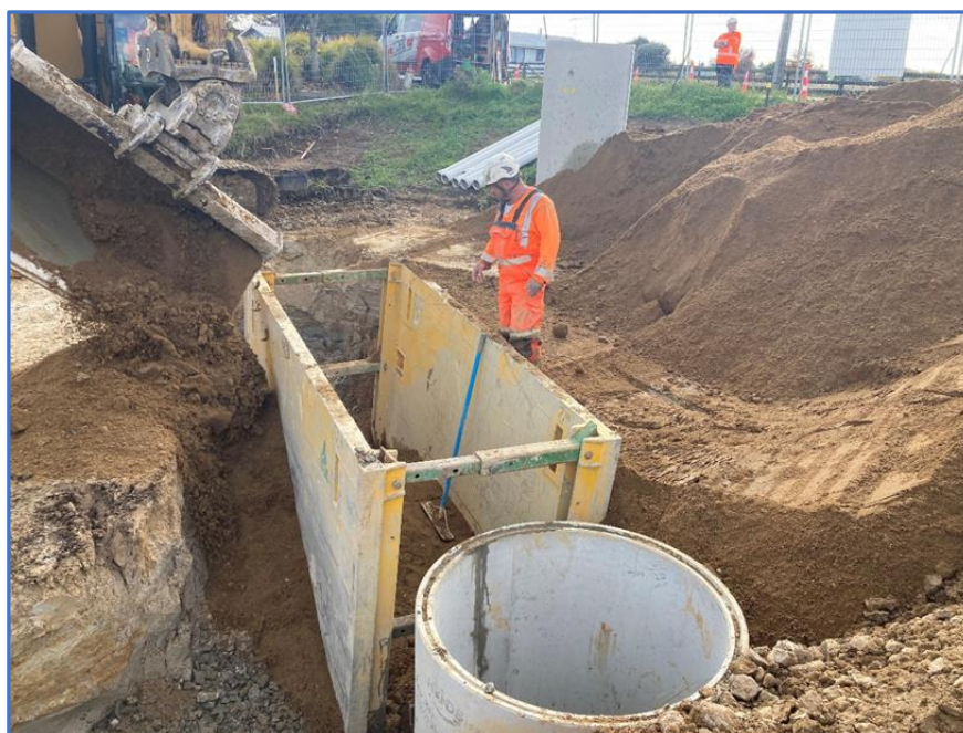
Construction of MH05 - Cambridge Road Site
