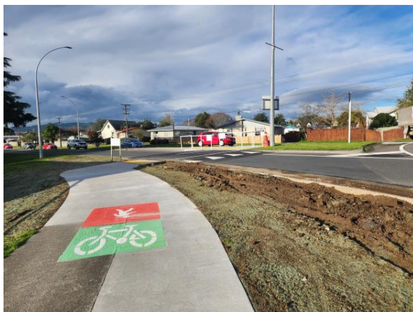
Figure 9: One vehicle space allowed before or after the Swedish-styled pedestrian crossing point on the northern approach of the roundabout
