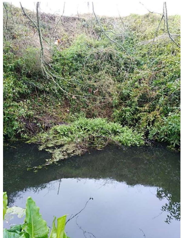
Photo 8: Submerged Culvert Outlet Under Cambridge Road
