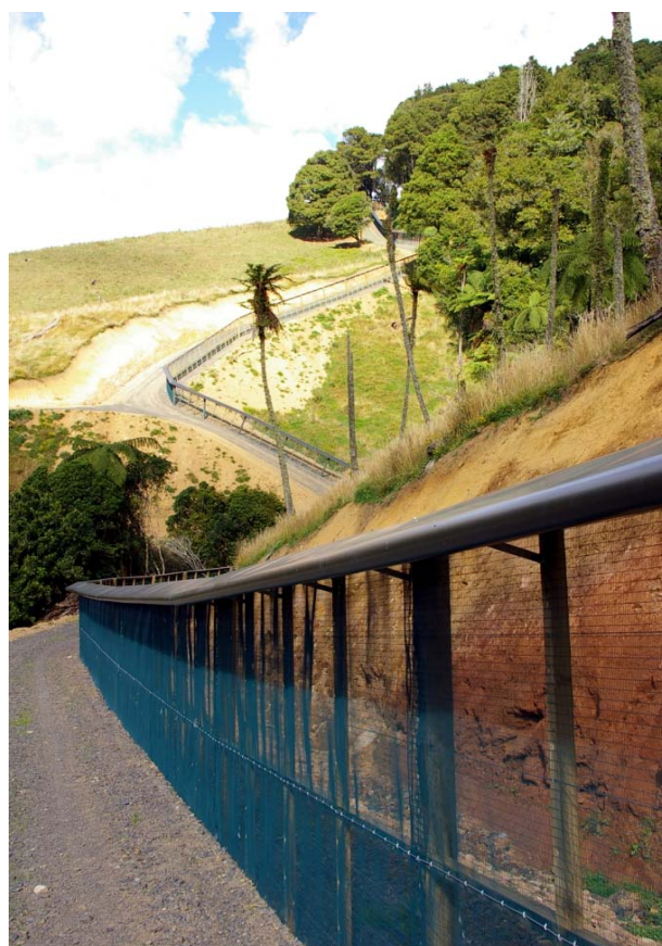
Completed pest-proof fence around Maungatautari Mountain
