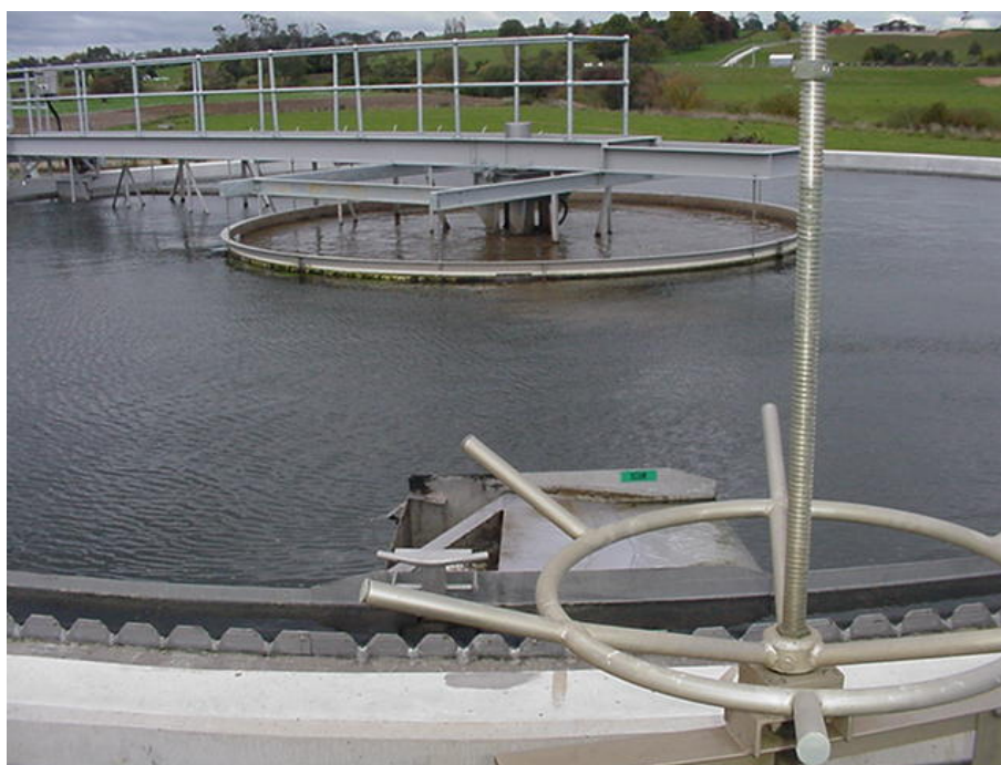
Te Awamutu Wastewater Treatment Plant
