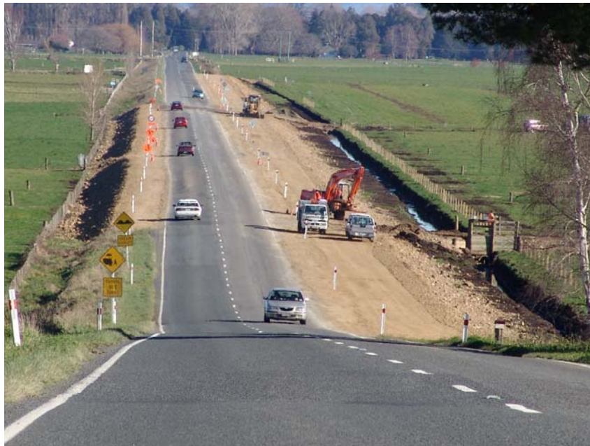
Rebuilding and resealing of Cambridge Road
