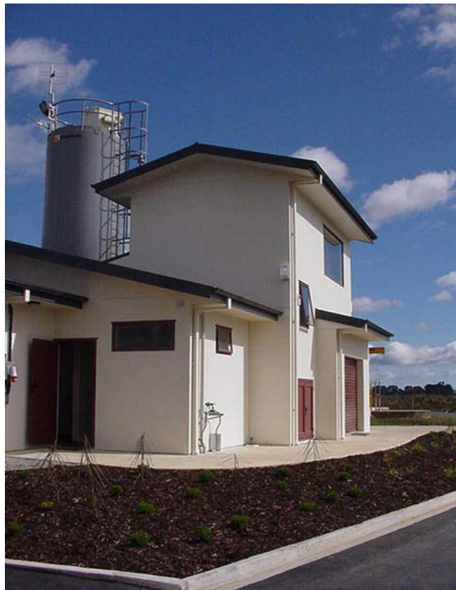
Wastewater Treatment Plant Te Awamutu
