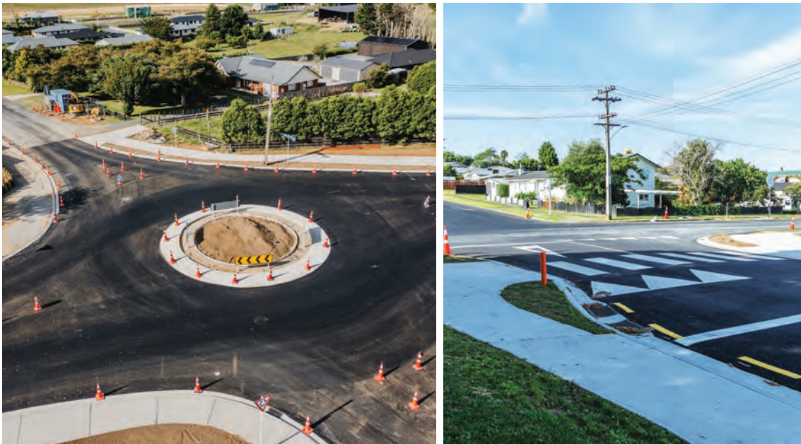
Te Ara Rimu, Kihikihi pathway under construction.
