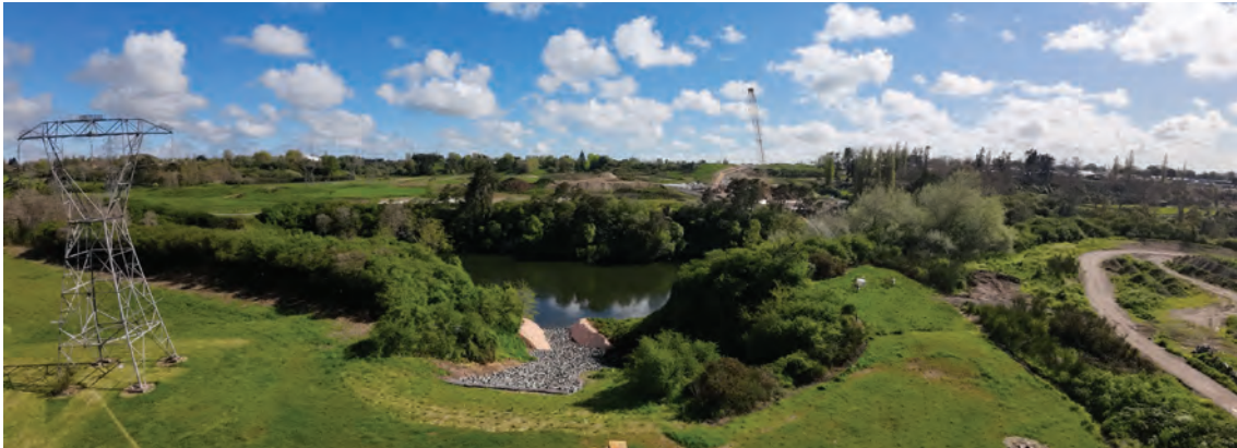
Cambridge Wastewater Treatment Plant outfall structure.
