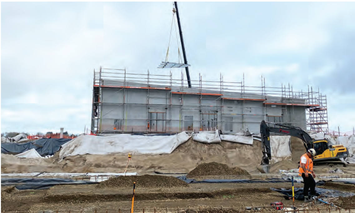
Cambridge Wastewater Treatment Plant construction.
