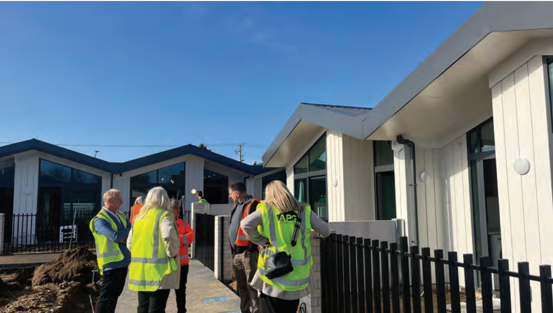
A place to call home for tenants at ten new pensioner housing units at Vaile Court in Leamington.
