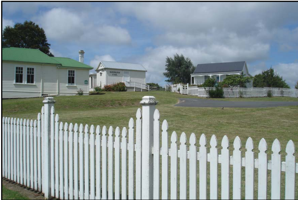
Figure 2: Old Police House (left) and Temple Cottage (right) Viewed from State Highway 3.
