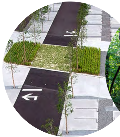
Multi-use Car Park Surface.
