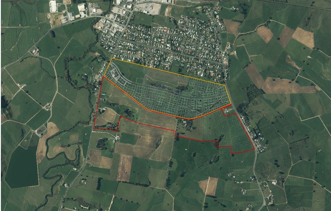
Figure 2: Aerial with site and immediate context 'Frontier Estate' to the immediate north of the site
