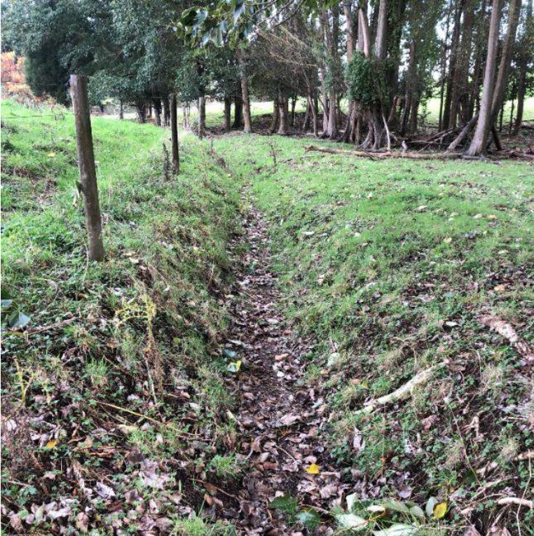
Figure 3 – Site outlet watercourse
