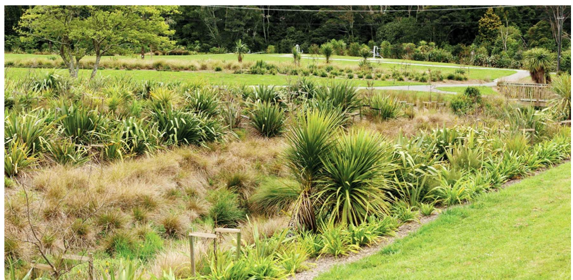
Figure 8– Planting swale example
