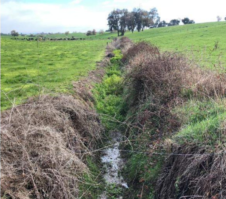
Figure 5 – Drainage channel below on-line pond.
