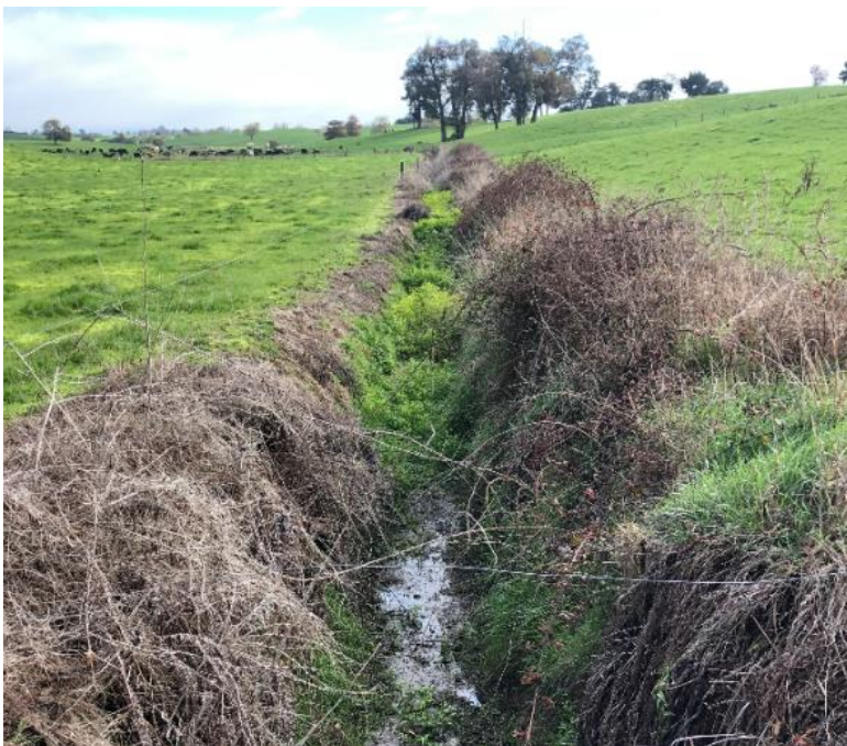
Figure 6 – Drainage channel below on-line pond.
