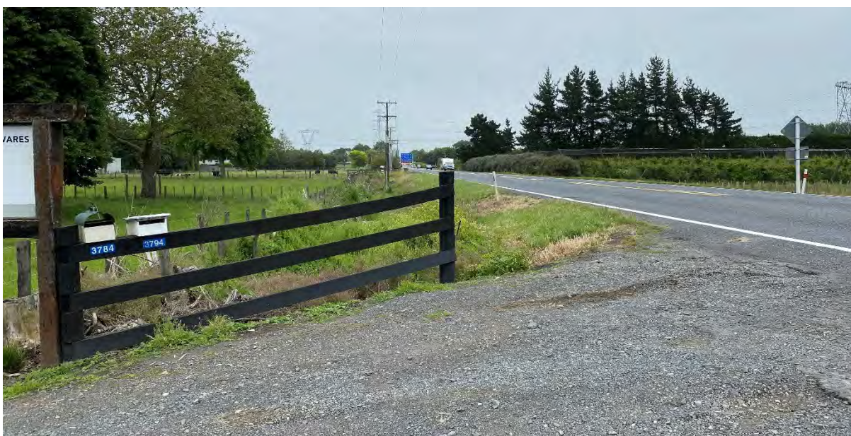
Figure 10: Sight distance from proposed intersection to the south
