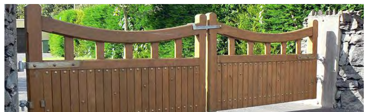
Timber farm style formal gate
