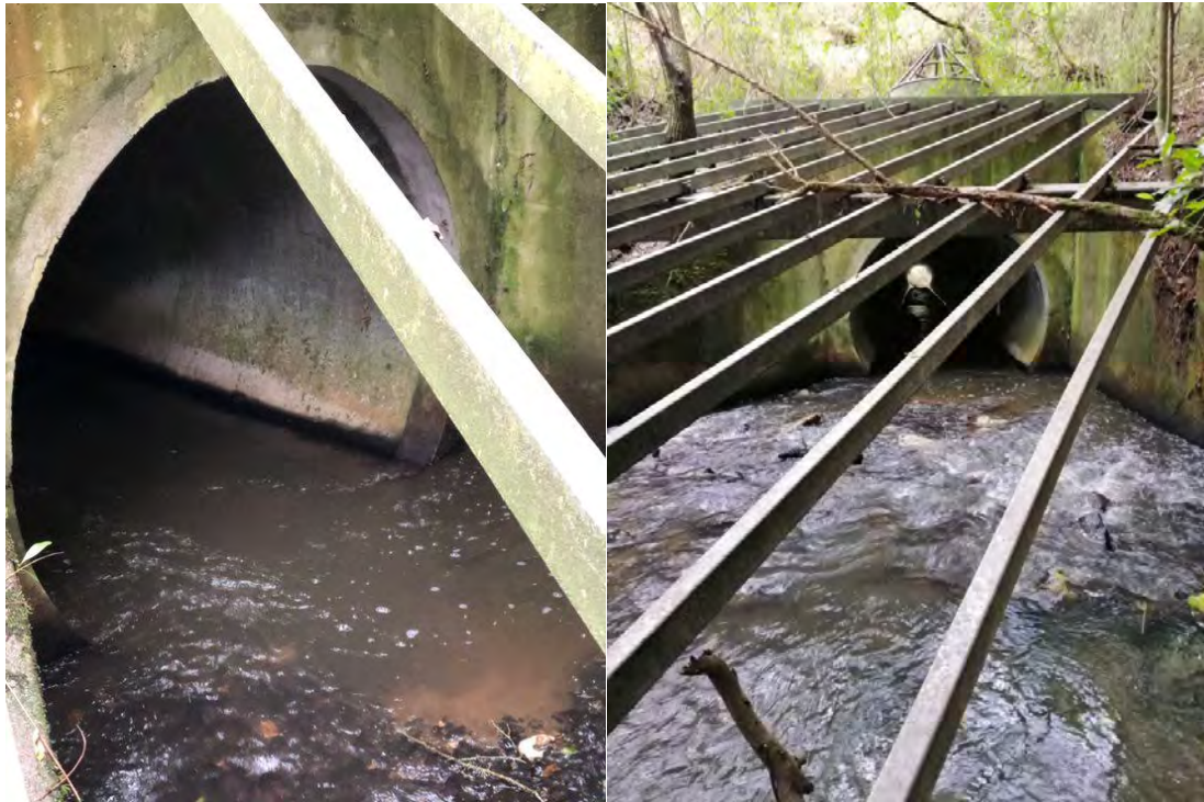
Figure 3-6: Culvert in the C4 Stream under Matos Segedin Drive.
