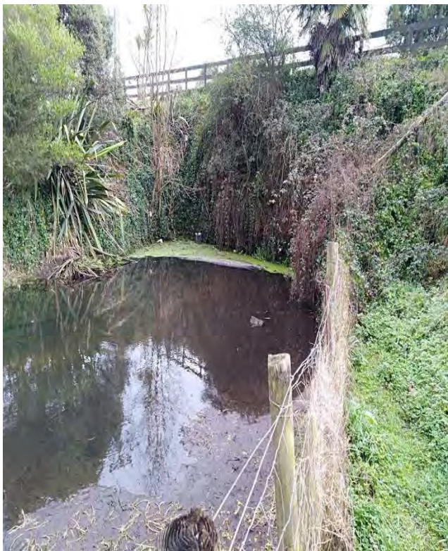
Photo 7: Submerged Culvert Inlet Under Cambridge Road
