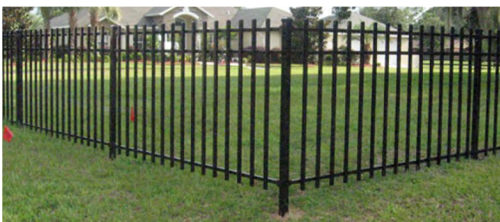
Visually permeable metal fencing
