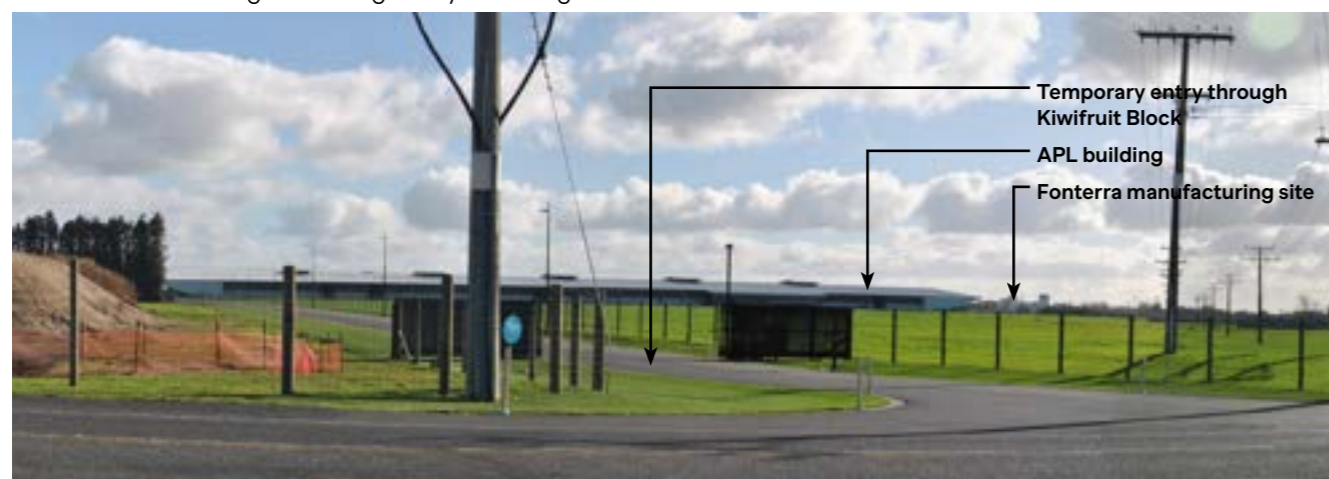
Figure 11 - Temporary entry to APL building, APL building, Fonterra Manufacturing Site and low voltage power lines.
