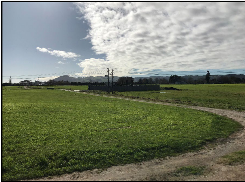
Photo 5: View from near the southern boundary of the site looking north towards the substation and the powerlines that run northwest to southeast across the centre of the site.
