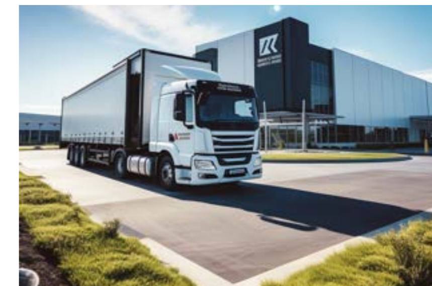
Design Guidelines encourage a high amenity environment for a wide range of industrial activity types.
