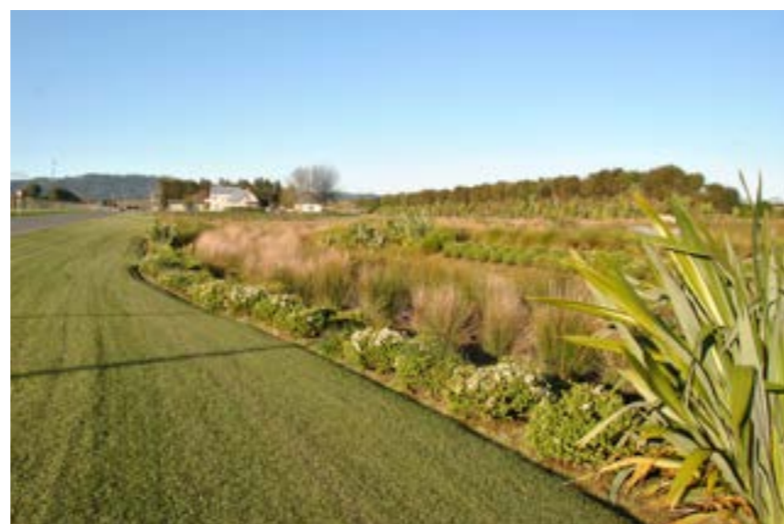
Recently constructed stormwater pond located in Bardowie Industrial Precinct.
