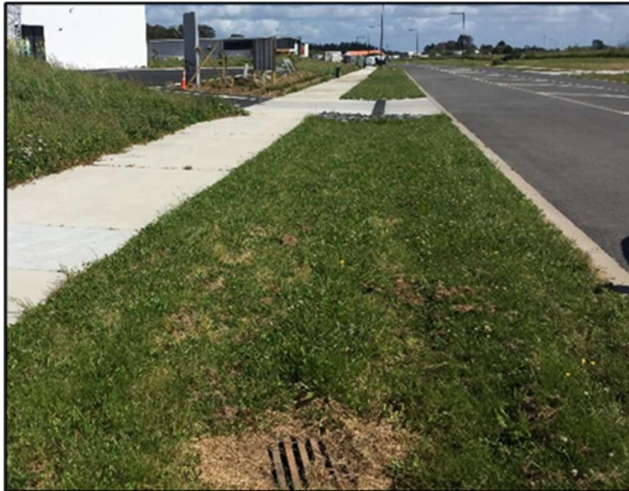
Figure 3 – Road Drainage System
