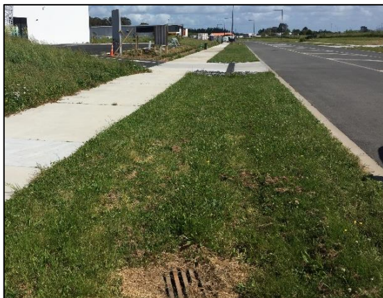
FIGURE 6: EXAMPLE OF STORMWATER SWALE AND SOAKAGE GRATE ALONG OSSIE JAMES DRIVE, CENTRAL PRECINCT
