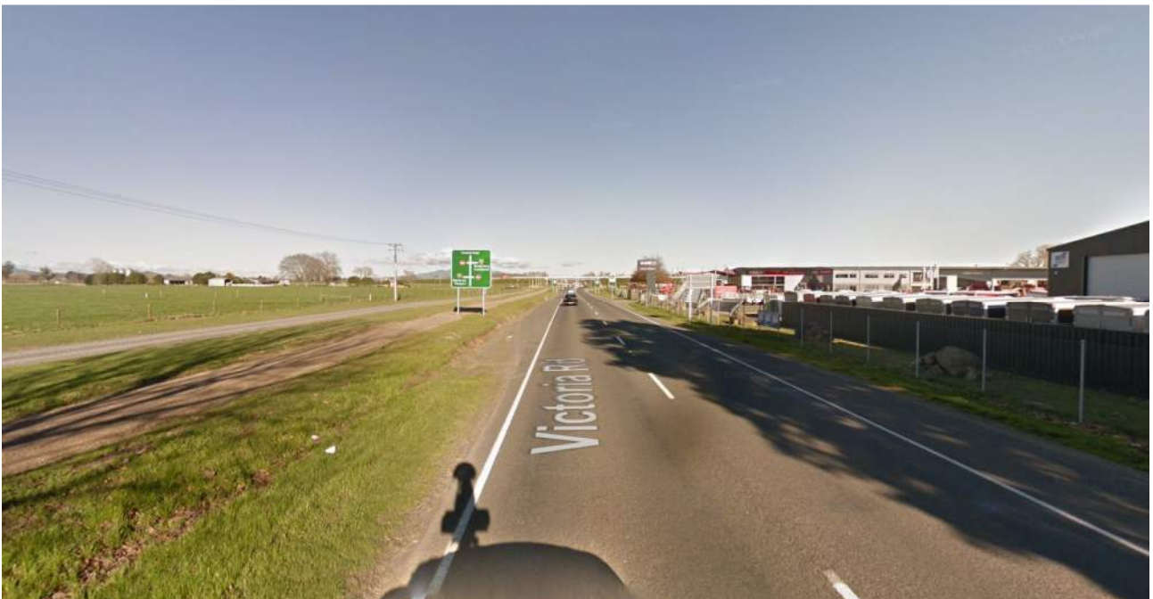
Figure 8: SH1B Victoria Road, south of Hautapu Road, looking South
