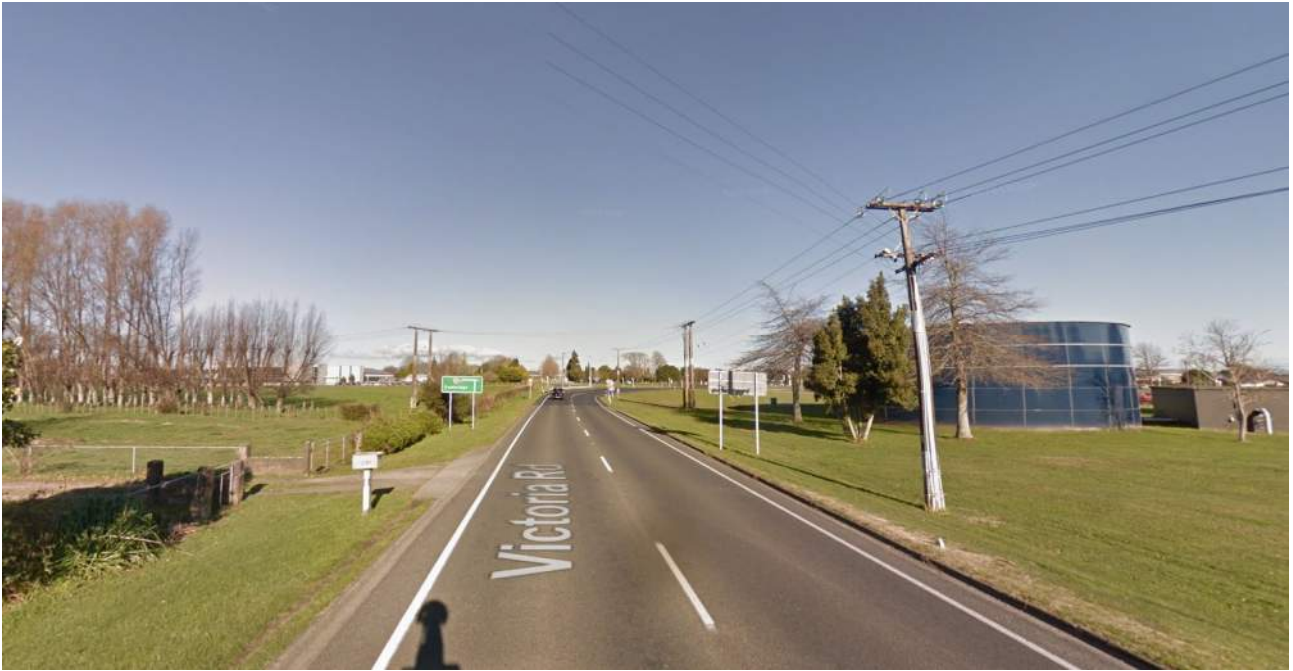
Figure 7: SH1B Victoria Road, north of Hautapu Road, looking South
