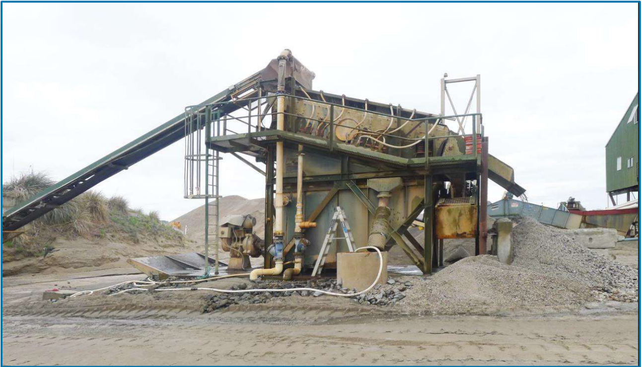
FIGURE 7: Screening Plant Example
