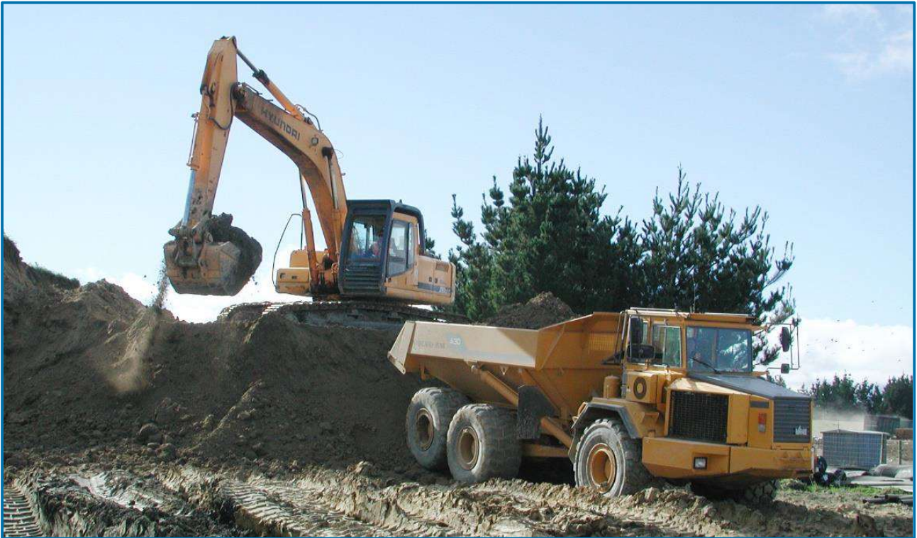
FIGURE 9: Excavator and Articulated Dump Truck Example
