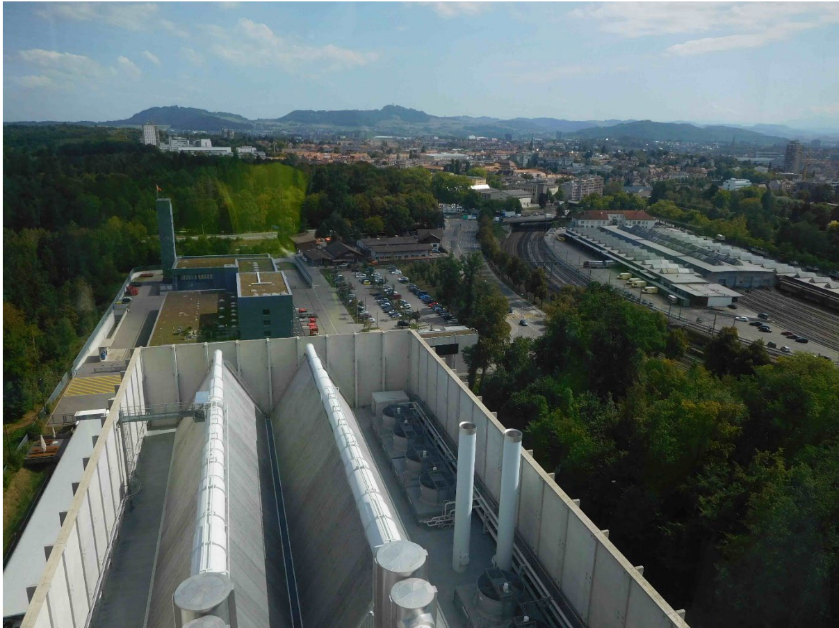
FIGURE 1 - VIEW FROM ROOF OF BERN WTE FACILITY LOOKING TOWARDS BERN CITY (BERN CITY FIRESTATION IN MIDDLE FOREGROUND – BLUE BUILDING)
