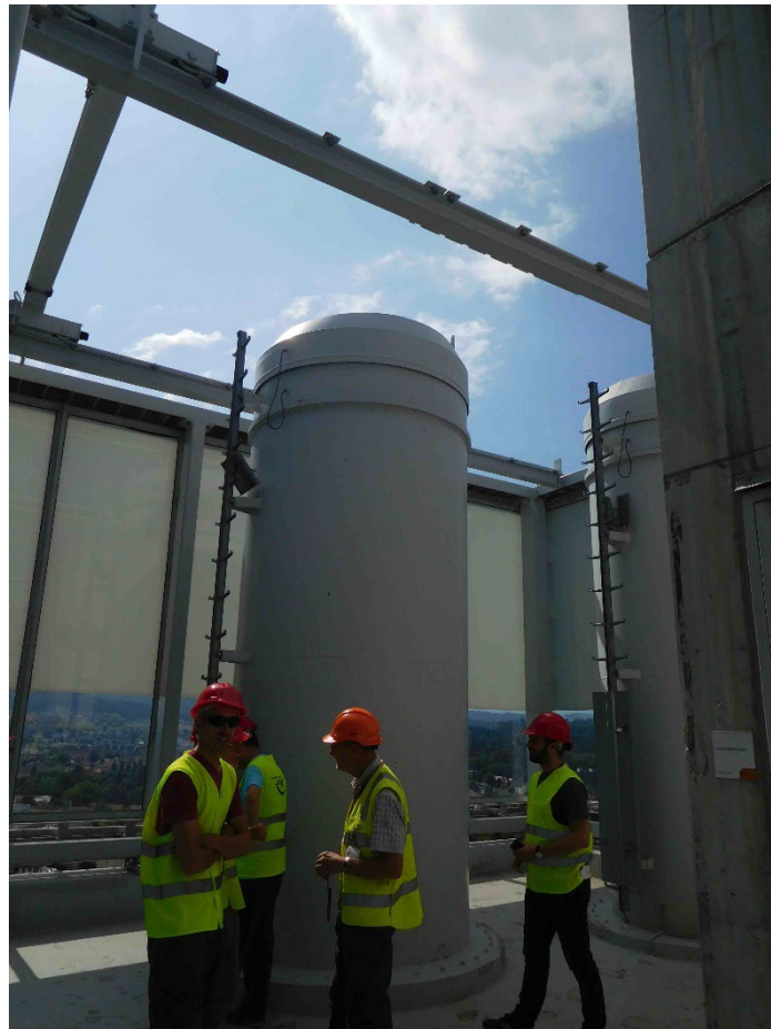
FIGURE 6 - BERN WTE PLANT CHIMNEY STACK: - NO SMOKE, NO SMELL; JUST HEAT
