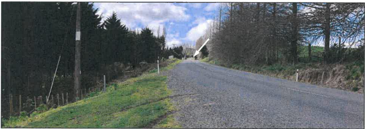
Figure 17: Looking north from Gate 3 (sight distance 250m – note arrow indicating location of red car emerging from sag vertical curve)
