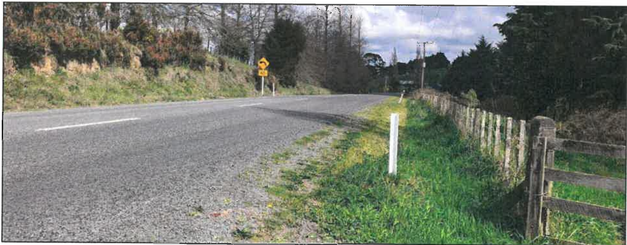
Figure 13: Looking south from the approximate location of Gate 2 (sight distance 220m)
