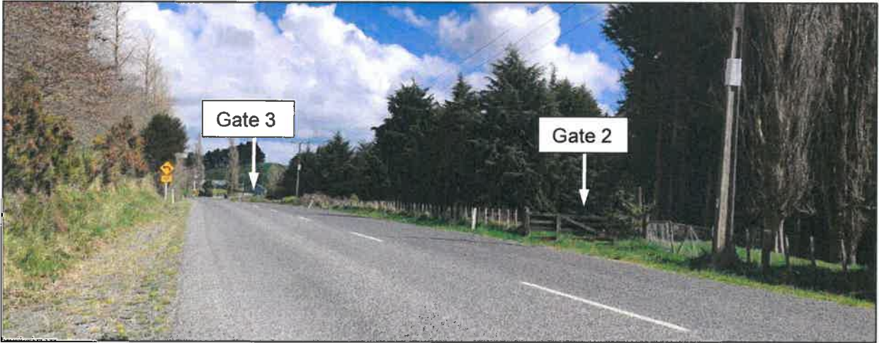
Figure 4: Existing frontage at the southern edge of the property looking south at the two existing vehicle crossings
