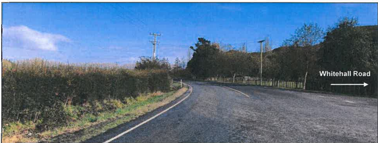
Figure 7: Looking west along Karapiro Road from Whitehall Road intersection (approx. location of a right-turning vehicle), showing approx. 115m sight distance.
