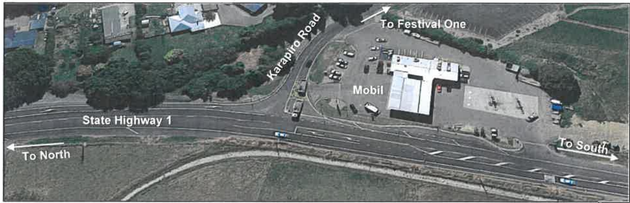
Figure 6: Intersection of State Highway 1 and Karapiro Road
