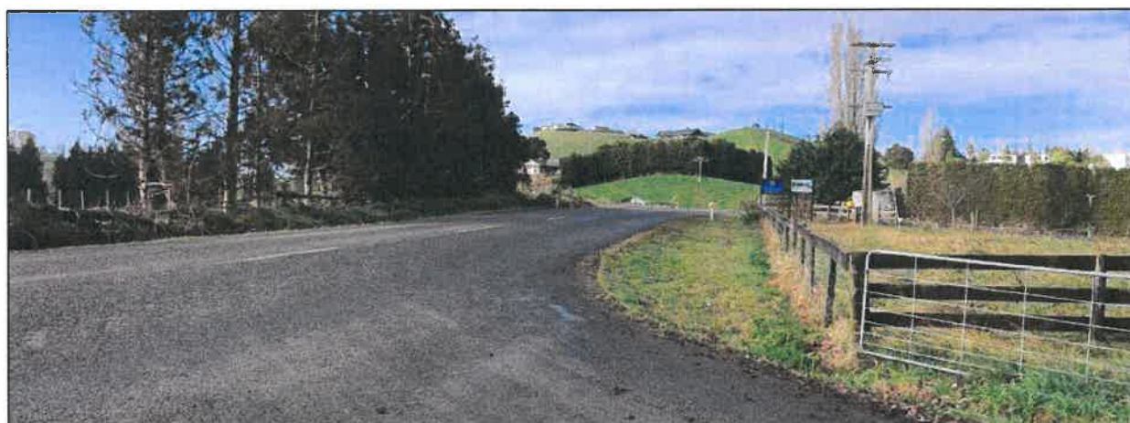
Figure 11: Looking south from the existing Gate 1 vehicle crossing (sight distance 122m)
