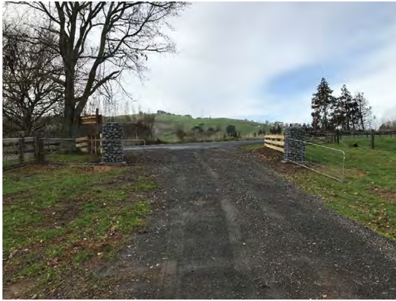
Figure 5: Site visit photo showing existing main entrance to the site (looking at Whitehall Road)
