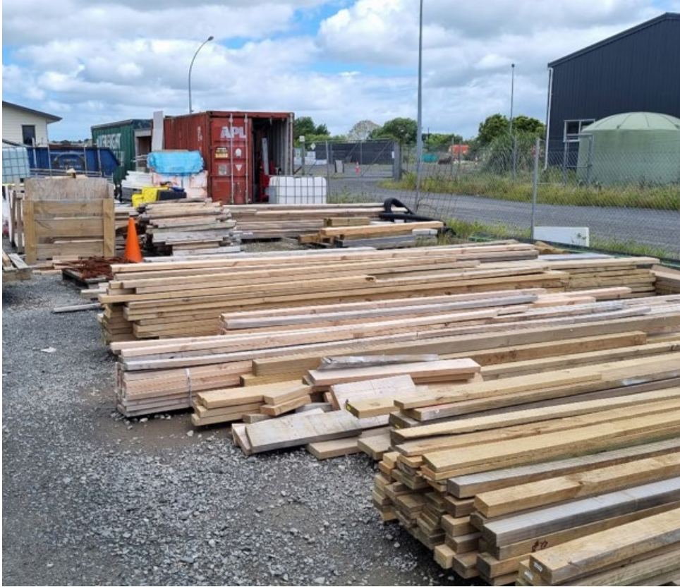
Photograph 5: Storage of potentially treated timber along northern boundary of the Kiwi Transportable Home's yard (Feature of interest 3).
