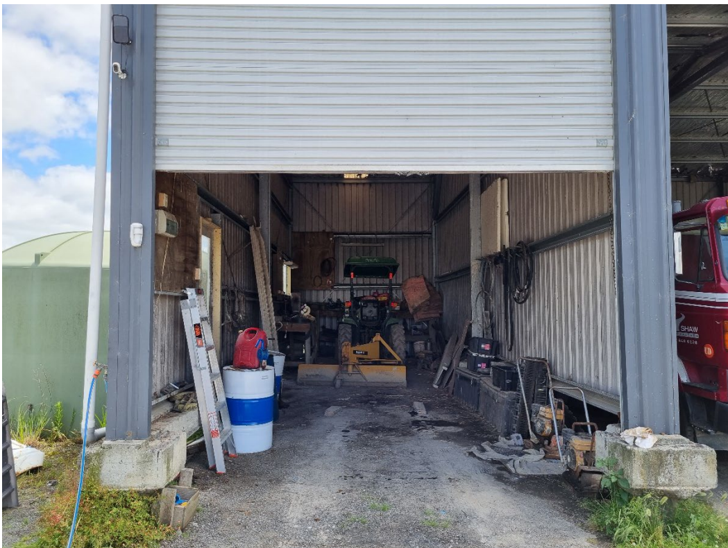
Photograph 20: 'Workshop' / storage shed on western boundary of Shaw Asphalters yard. Numerous black stains on ground. 2 x 200 L steel drums of kerosene and 1 x 200 L steel drum of hydraulic fluid (Feature of interest 15).
