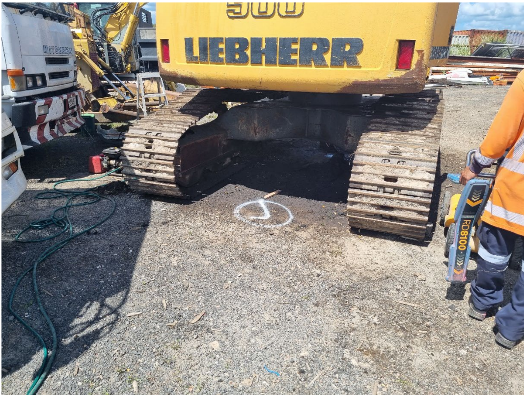
Photograph 14: Staining of ground surface beneath excavator in Pro Demolition yard (Feature of interest 10).
