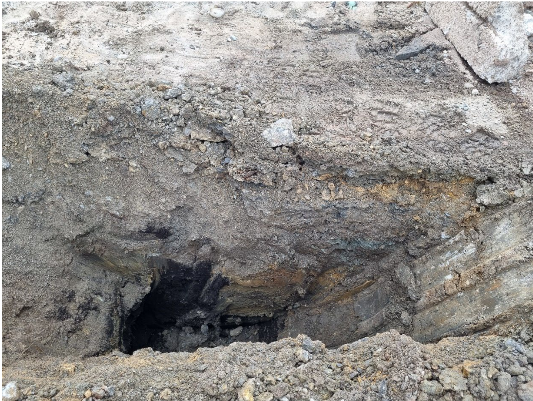
Photograph 26: Typical mixed fill encountered across the investigation area. Note the black peat at the bottom of the test pit.
