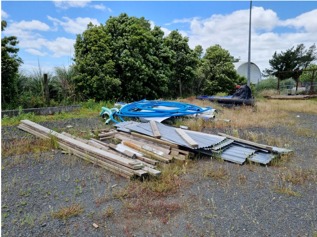
Photograph 15: Small pile of uncovered timber in the Cambridge Construction yard (Feature of interest 11).
