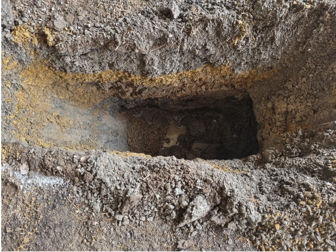
Photograph 25: Compacted layers of gravel and coarse-grained sand as observed at TP08.
