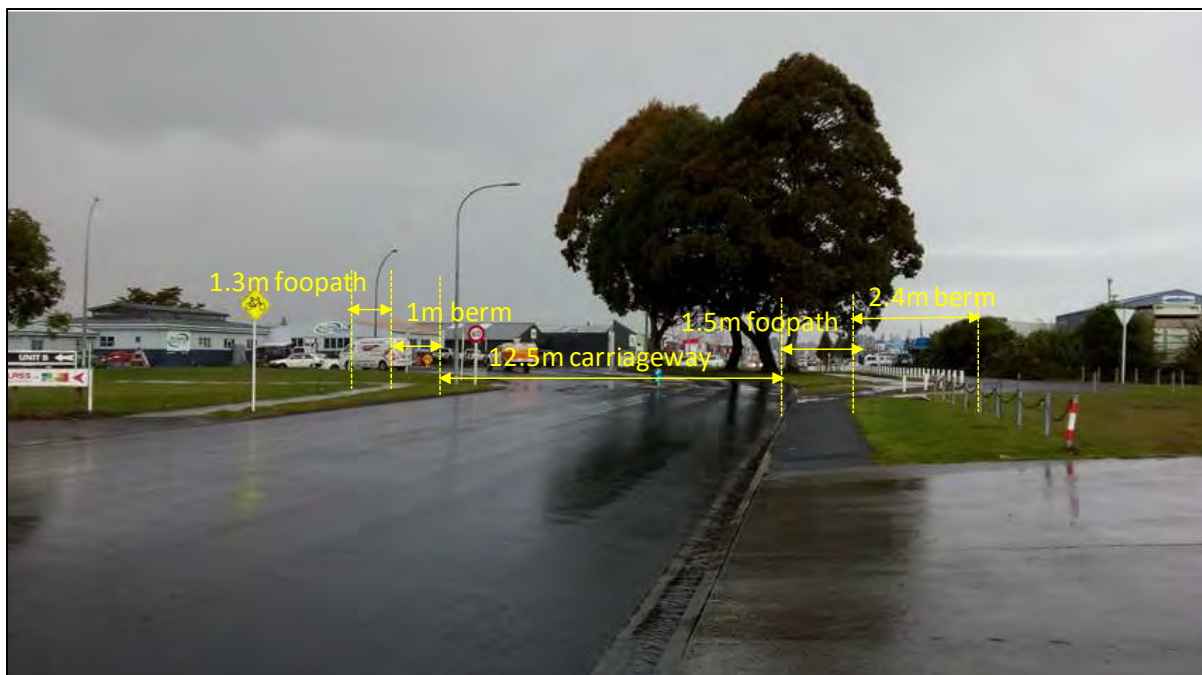
Figure 7: Kahikatea Drive Cross Section
