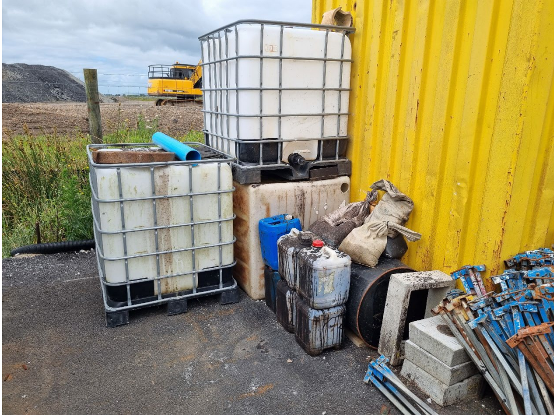
Photograph 1: Empty IBCs, 20L plastic containers (part filled with unknown black liquid (possibly bitumen emulsion)) and empty 200 L steel drum in far southeast yard of the site (Feature of interest 1).
