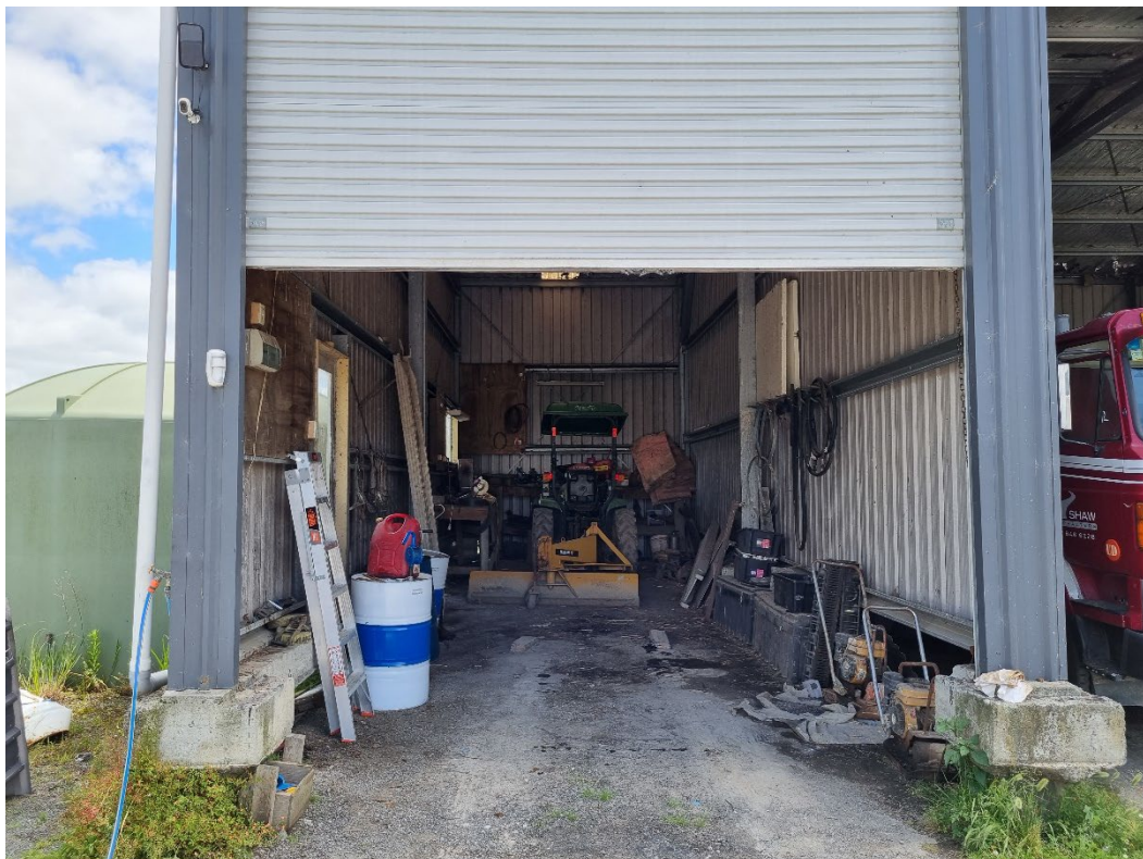
Photograph 20: 'Workshop' / storage shed on western boundary of Shaw Asphalters yard. Numerous black stains on ground. 2 x 200 L steel drums of kerosene and 1 x 200 L steel drum of hydraulic fluid (Feature of interest 15).
