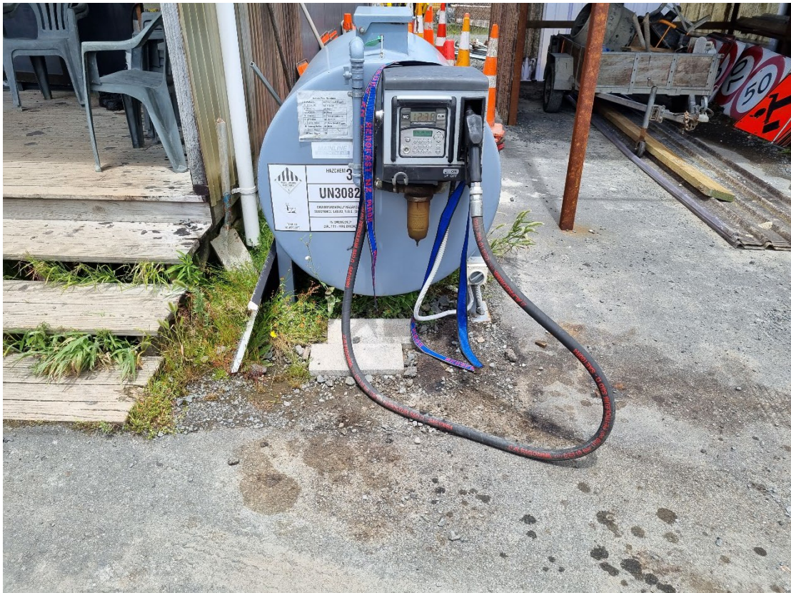
Photograph 16: Un-bunded diesel AST in Shaw Asphalters yard (central north of the site) (Feature of interest 12).
