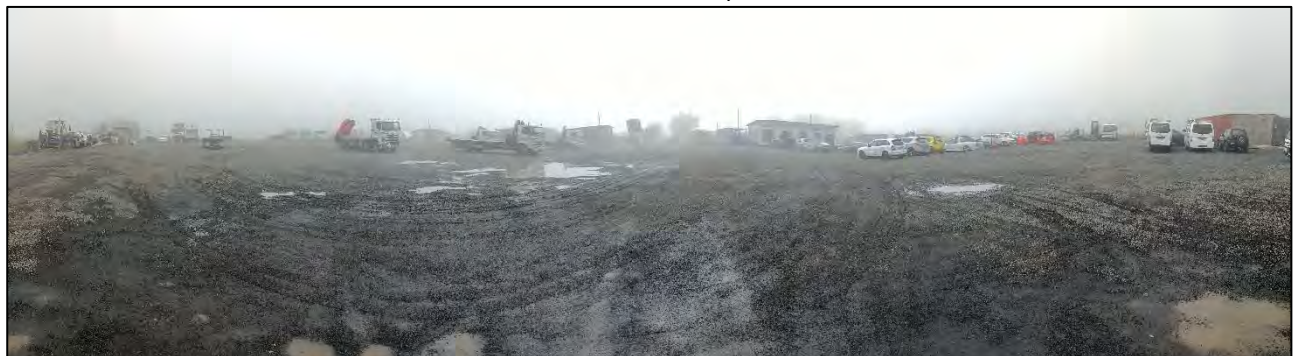
Figure 5: Site visit photo from the southern boundary facing northwards showing the existing activities that operate on the subject site
