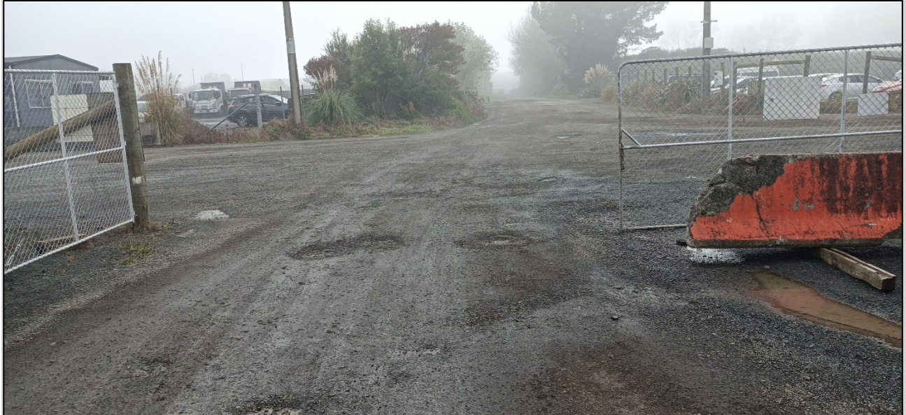
Figure 7: Site visit photo from the entrance of the subject site looking northward down the existing accessway.
