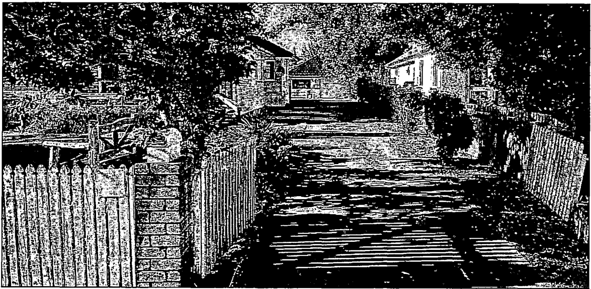
Figure 4: Site visit photo showing existing access to the site
