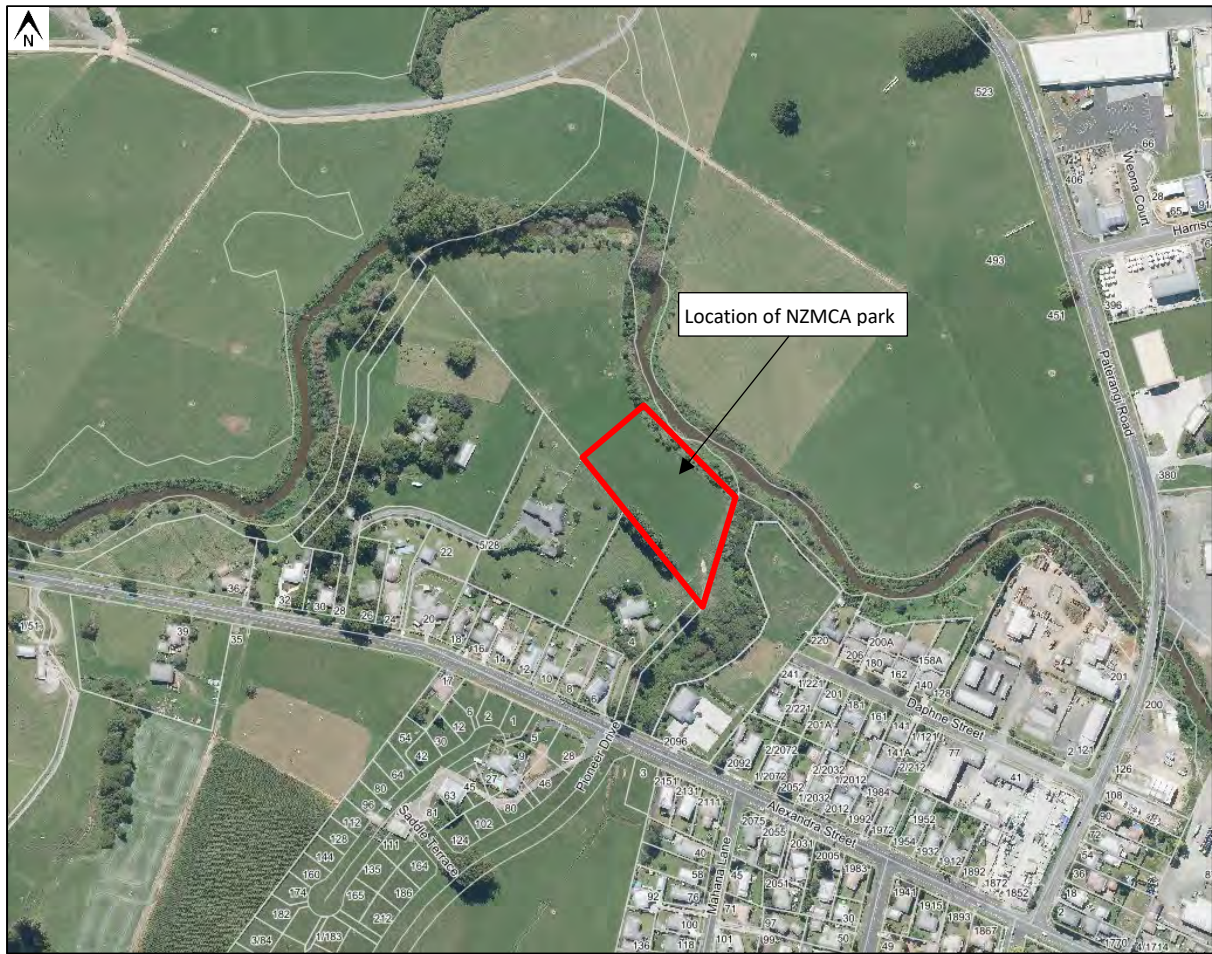
Figure 1: shows the location of the NZMCA park located in Pirongia.
