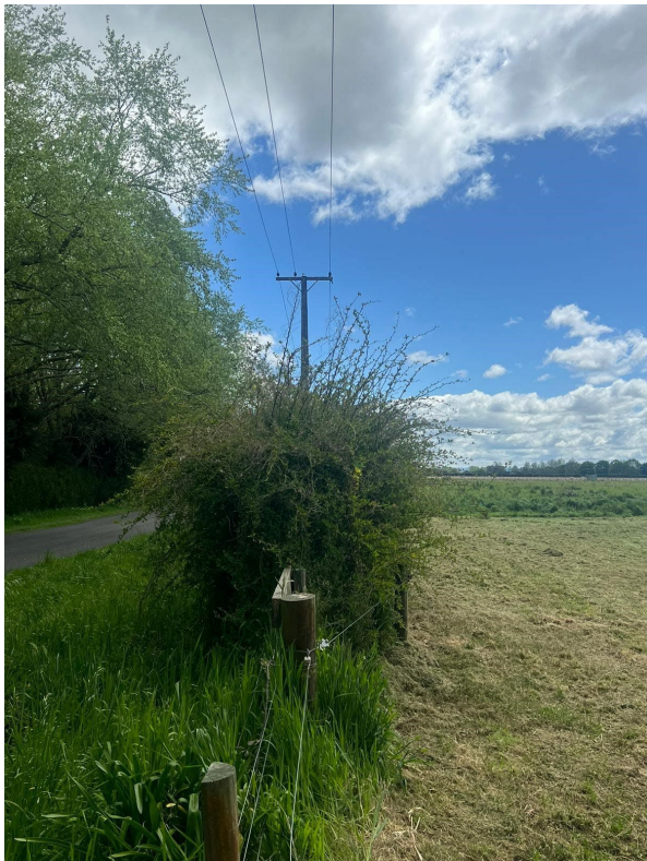
Figure 5: Sites frontage with Parallel Road (western side of site) illustrating existing barberry hedging, to be replaced with Cryptomeria shelterbelt – the overhead powerline in this location only has one 11kv line
