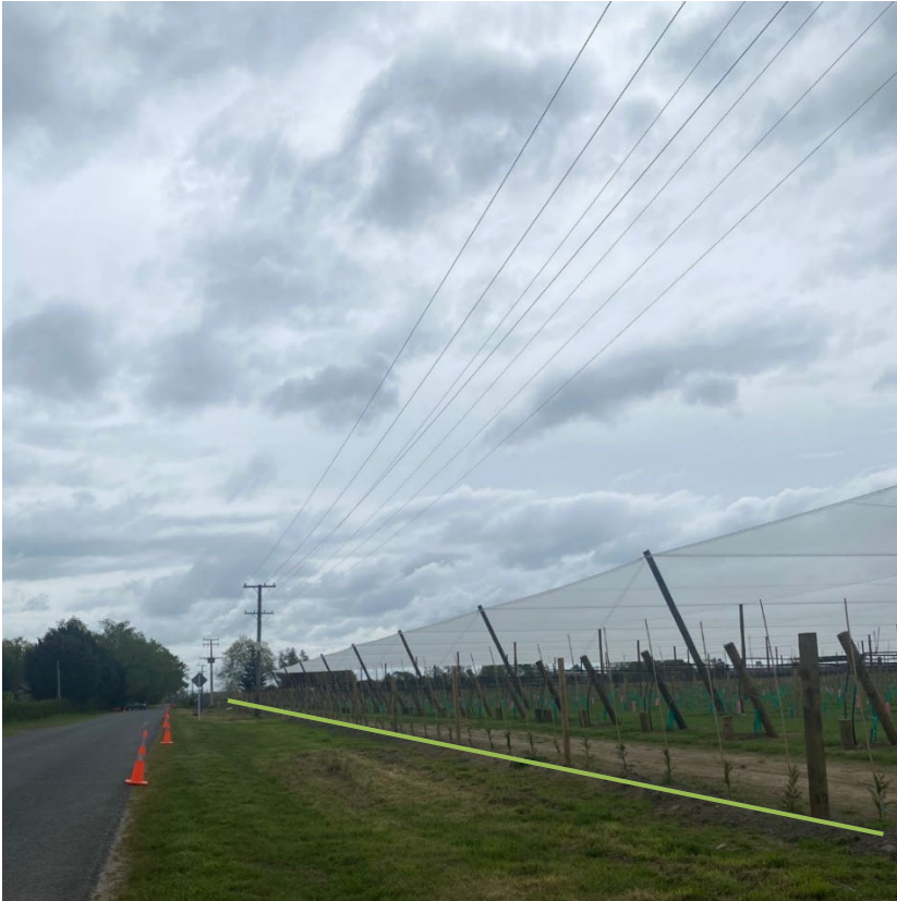
Figure 5: Site visit photo showing recently planted shelterbelts looking west along the eastern portion of Parallel Road, green line indicates the location of the base of the plants with the 11kv and 400v powerlines directly overhead.
