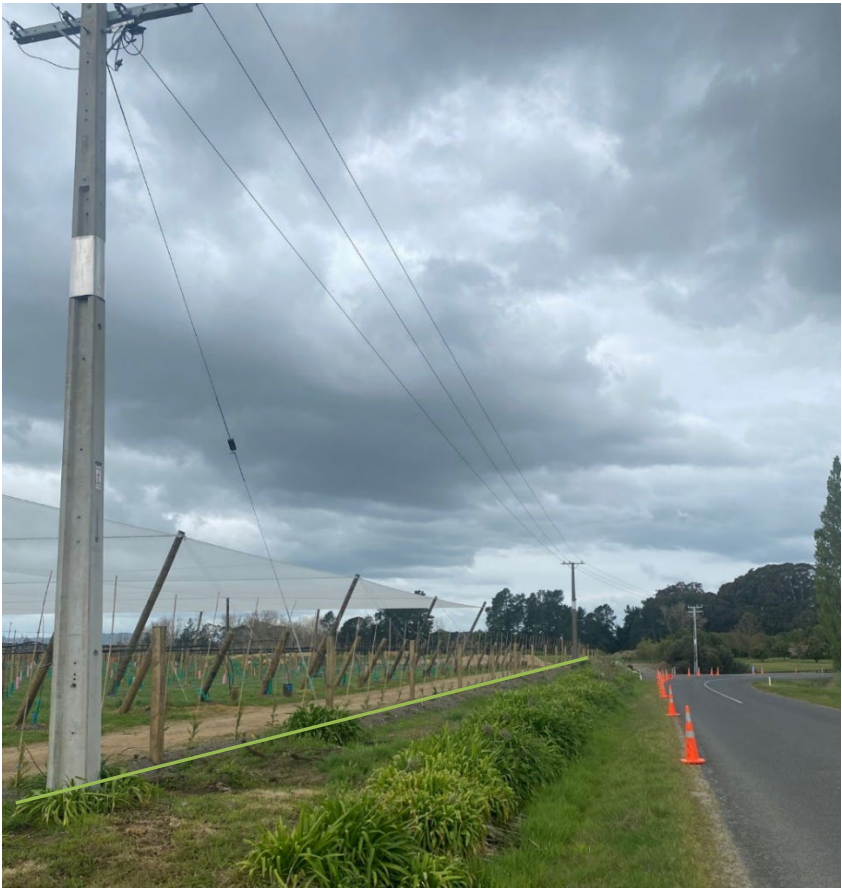
Figure 6: Site visit photo showing recently planted shelterbelts looking east along the eastern portion of Parallel Road, green line indicates the location of the base of the plants with the 11kv powerlines directly overhead.
