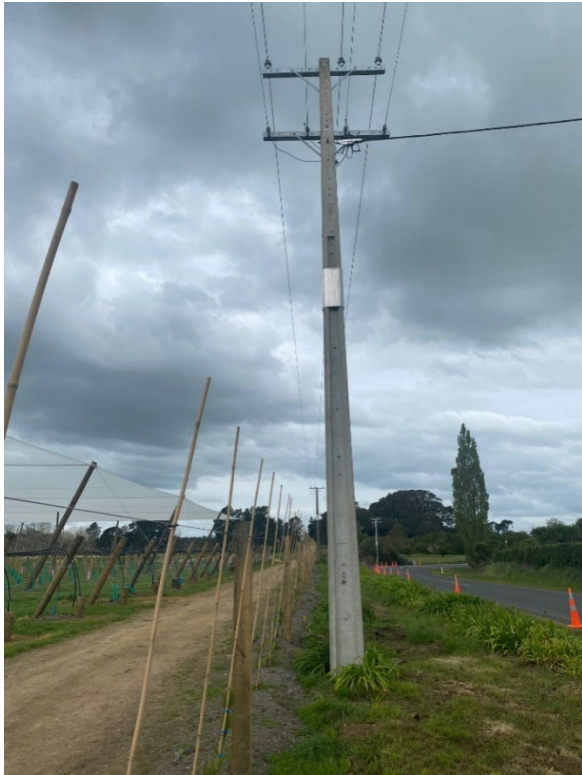
Figure 7: Site visit photo showing the plants proximity to the lines.
