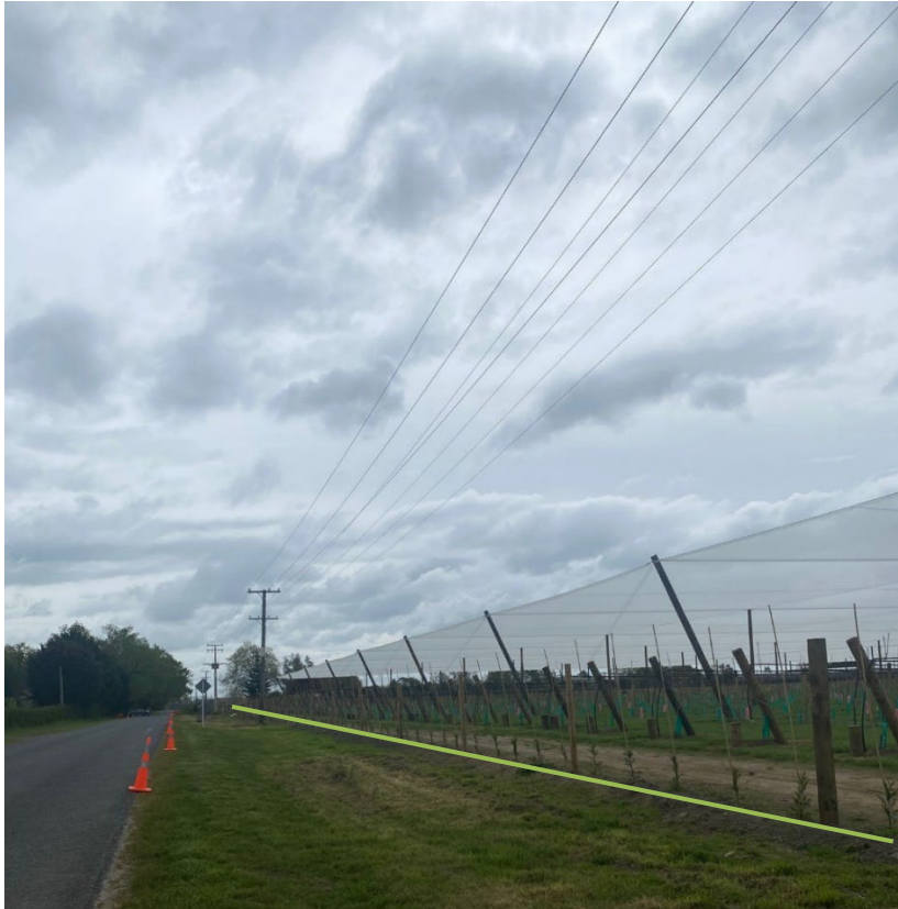
Figure 5: Site visit photo showing recently planted shelterbelts looking west along the eastern portion of Parallel Road, green line indicates the location of the base of the plants with the 11kv and 400v powerlines directly overhead.
