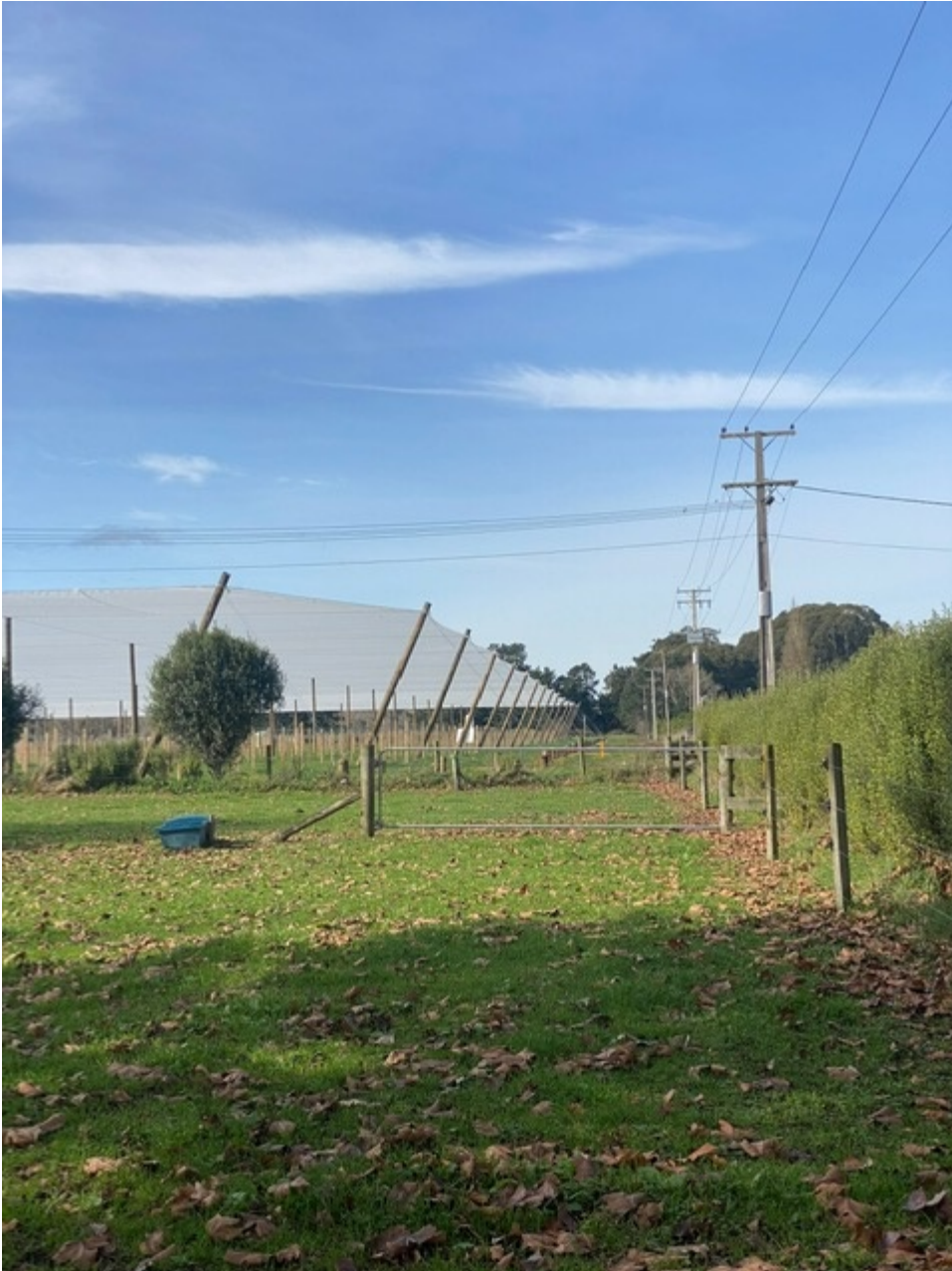
Figure 7: Site visit photo showing the shelters back from Parallel Road (Parallel Road on the right hand side, from inside the boundary of 598 Parallel Road).
