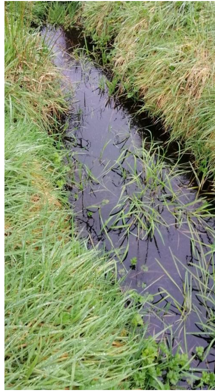
Figure 5: Standing water present upstream of the culvert.
