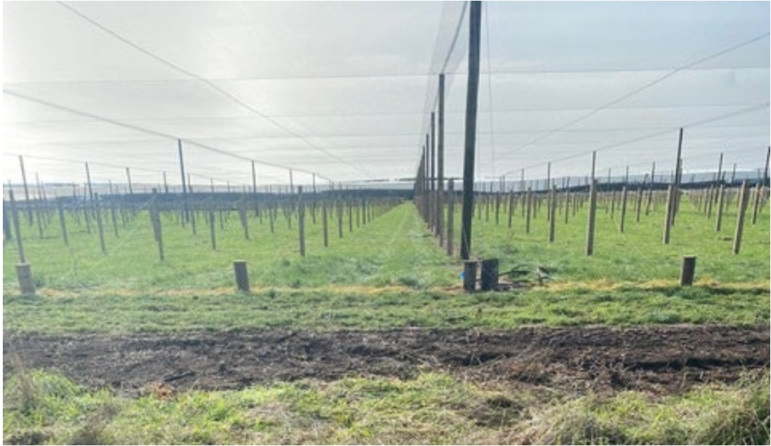
Figure 6: Site visit photo showing the shelters stretching back from Parallel Road.
