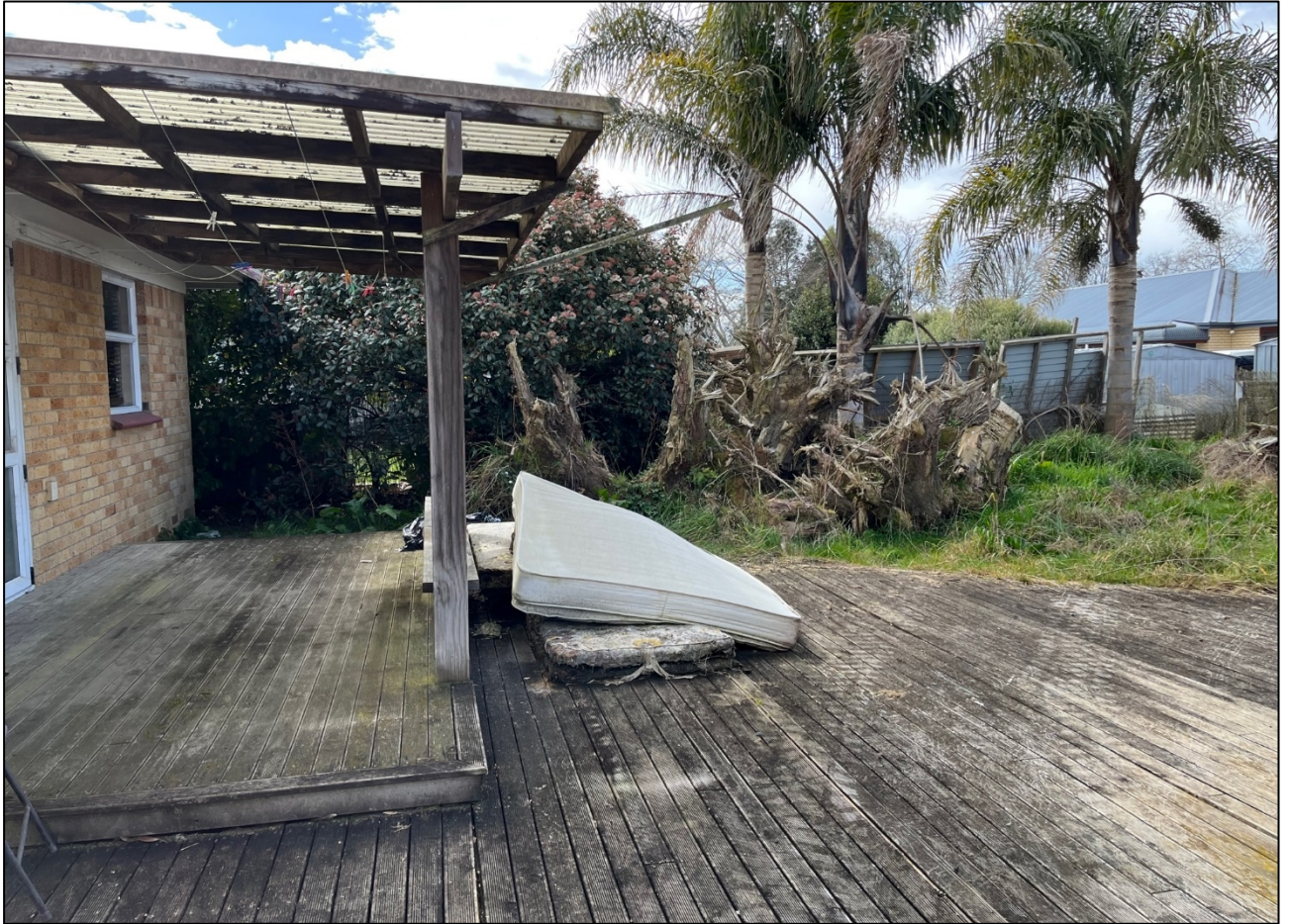
Figure 9: Site visit photo showing rear of existing dwelling facing 5 Kelly Road.
