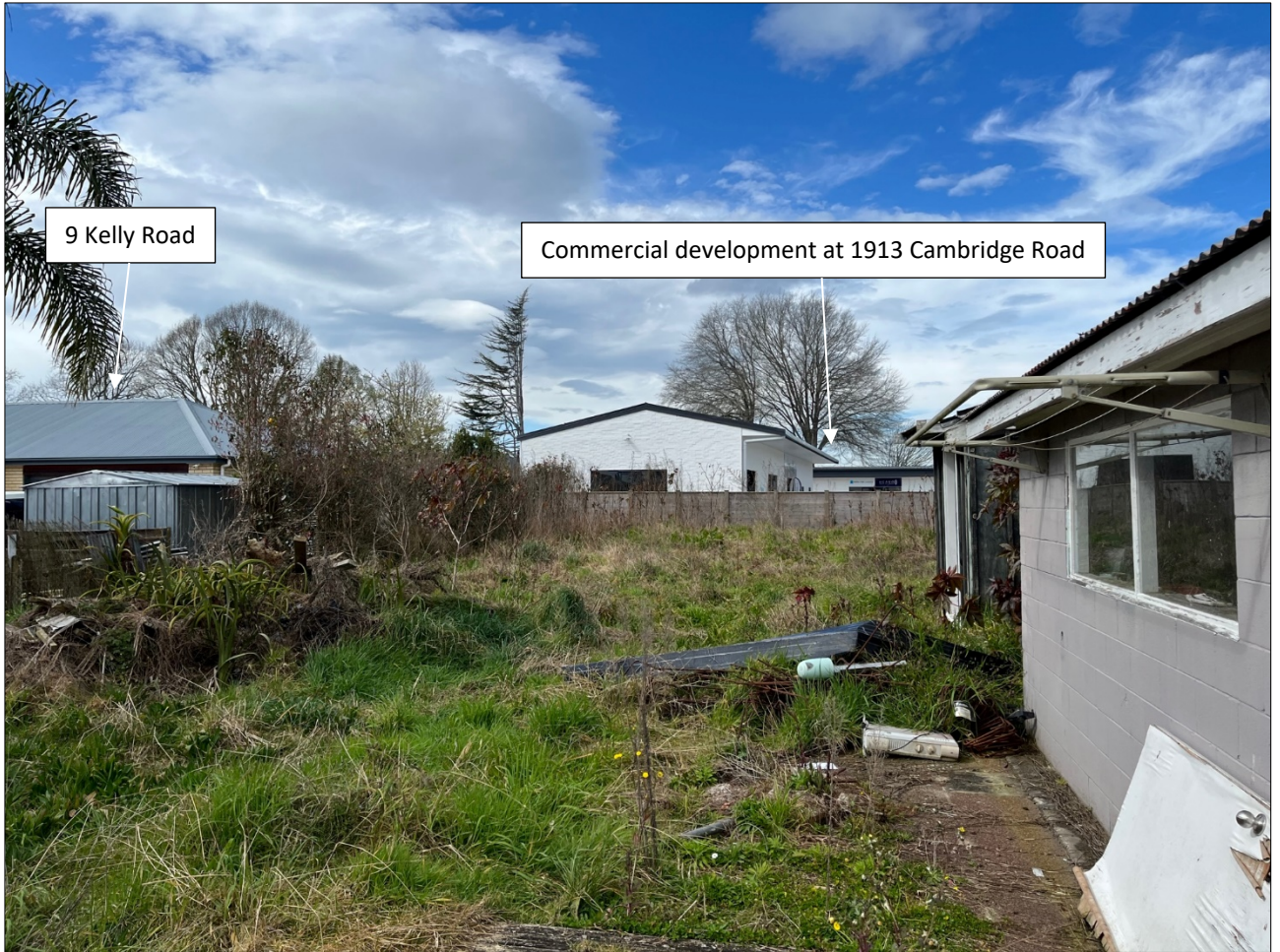
Figure 10: Site visit photo showing rear of the site facing east towards commercial development.
