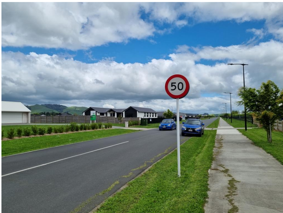
Figure 7: View of an existing street in the subdivision showing sight distance
