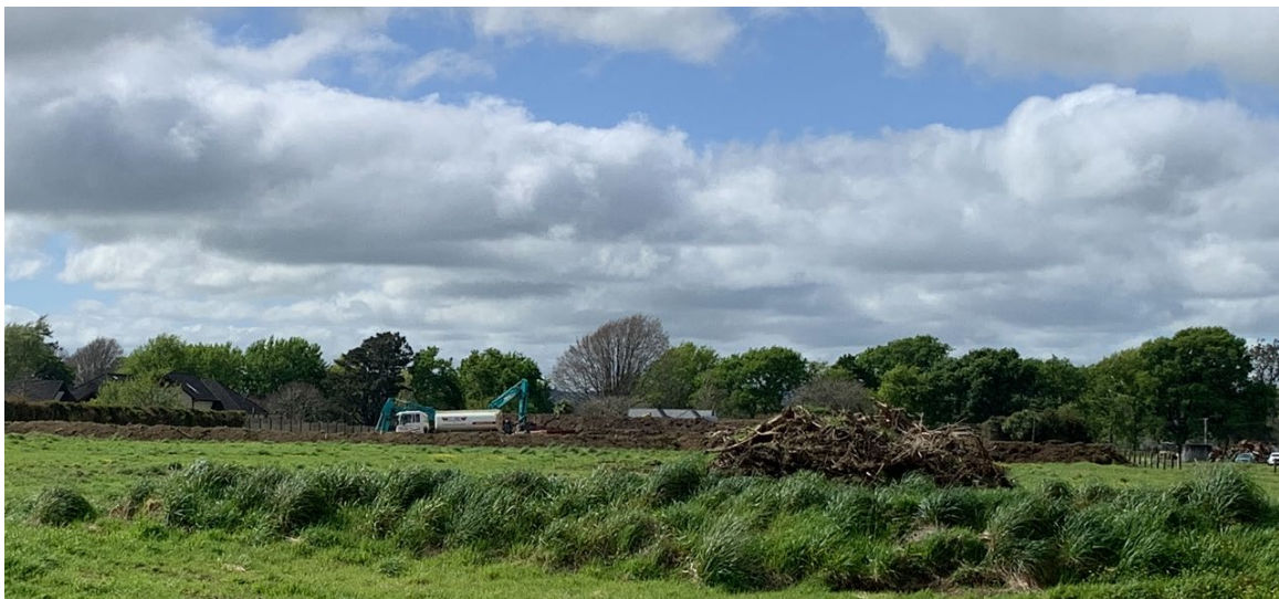
Earthworks around the rubbish pit area
