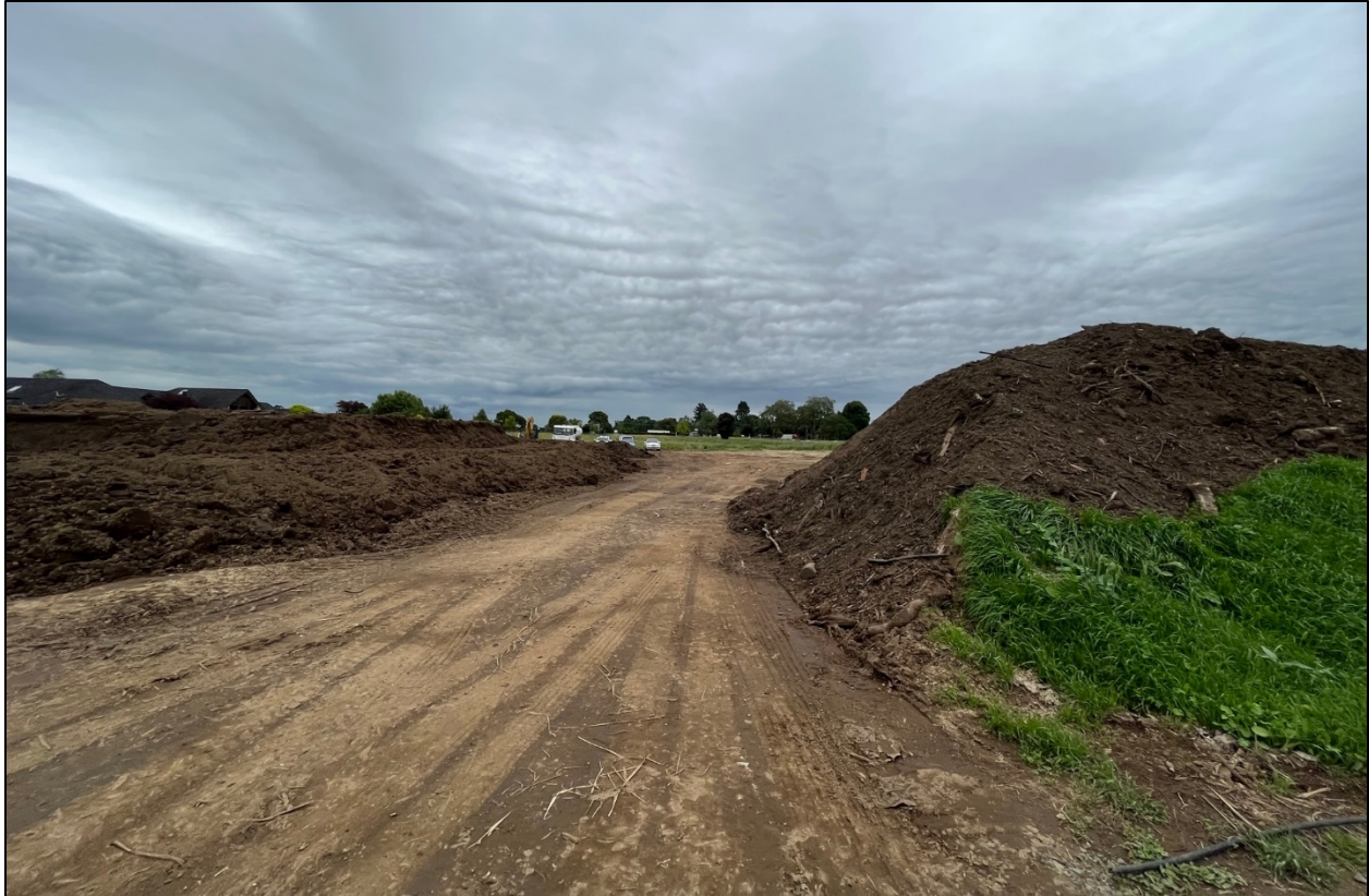
Figure 17: Site visit photo showing earthworks on site.
