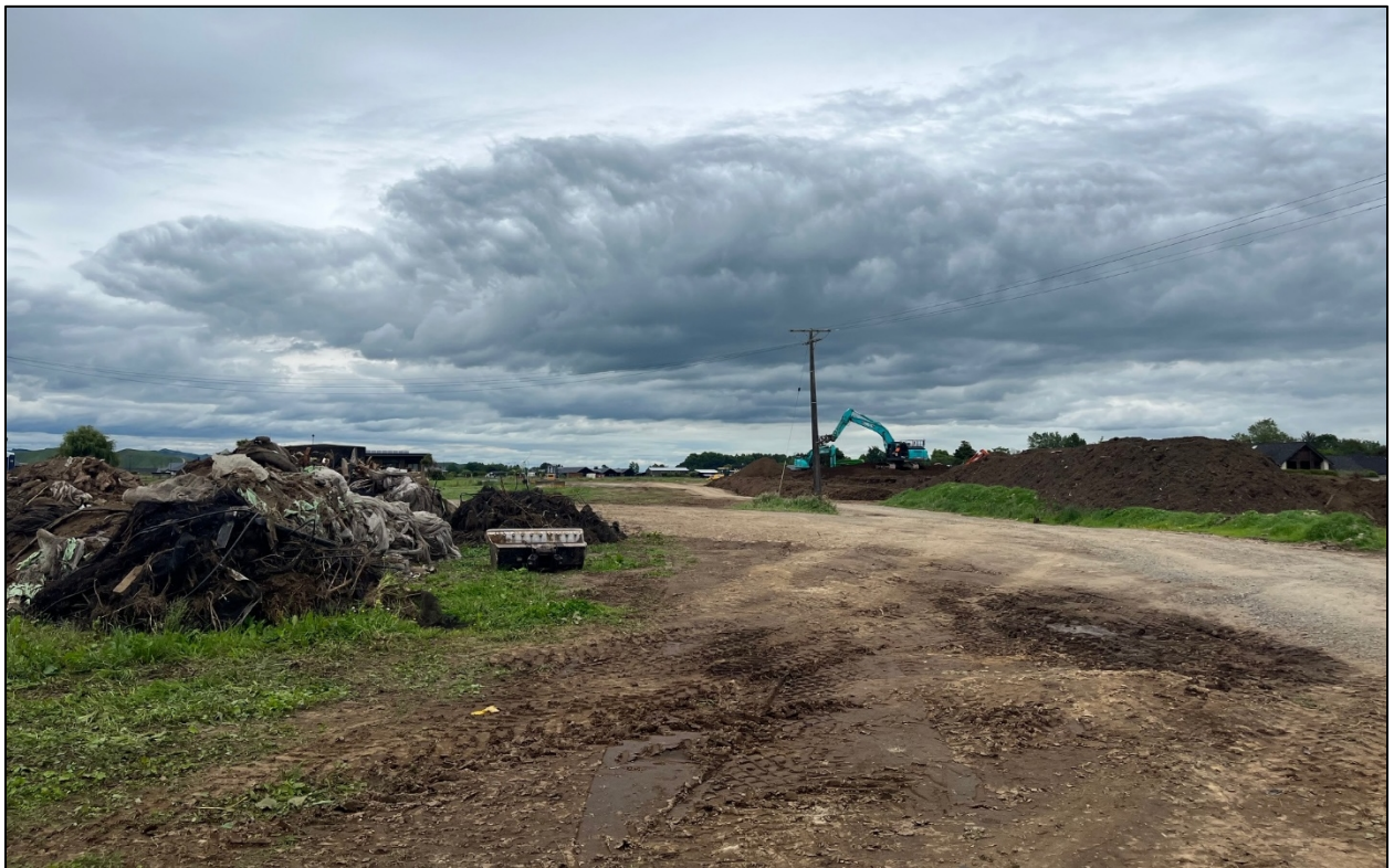
Figure 10: Site visit photo showing Lot 11.
