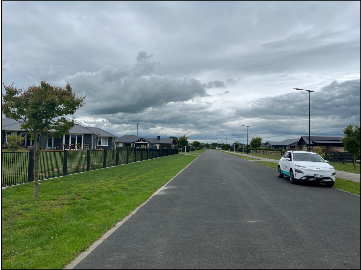
Figure 23: Site visit photo showing down existing road of Te Mara Drive.
