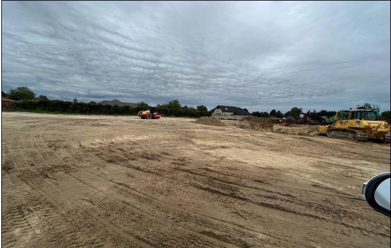
Figure 15: Site visit photo showing neighbouring properties.
