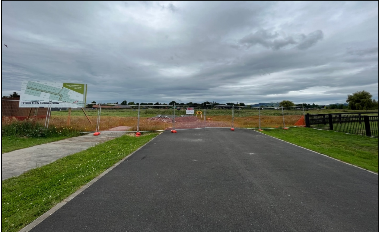
Figure 21: Site visit photo showing end of Te Mara Drive where new road/Lot 200 will start.
