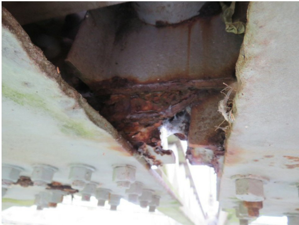
Figure 6-2 – Central Pin Original Construction Details
